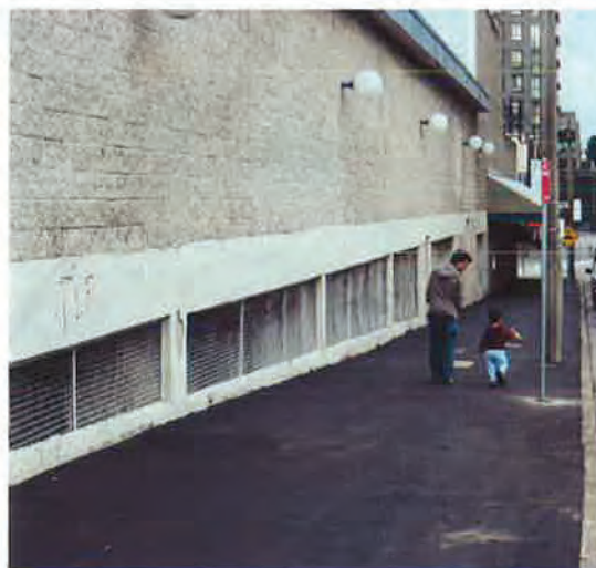
UNDESIRABLE: Inactive street frontages poor pedestrian environment, little passive surveillance of street, poor public-private domain interface, and little reason to spend time in this area
