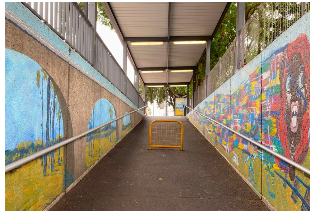
Ramp heading north, on the western side of the rail line. Mural is on both sides of the ramp. The roof covering the ramp reduces lighting, however, this side of the tunnel is brighter likely due to the brighter coloured murals, the lack of landscape between the footpath and the ramp and the western aspect.
