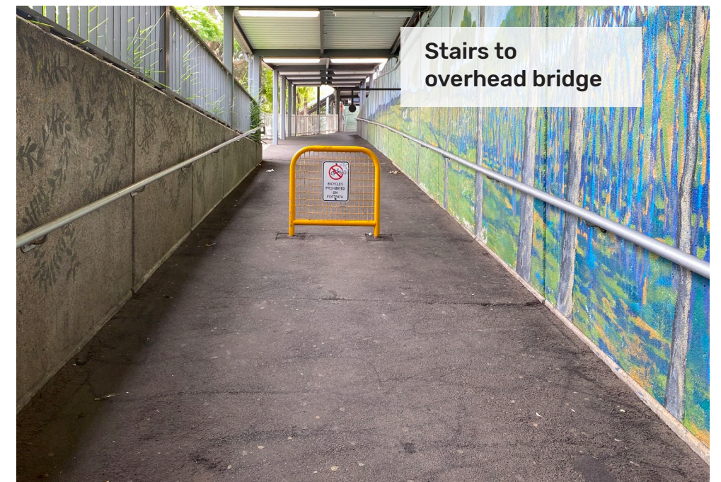
Views up ramp. Beyond is another ramp that leads to the overhead pedestrian bridge and platform access.
