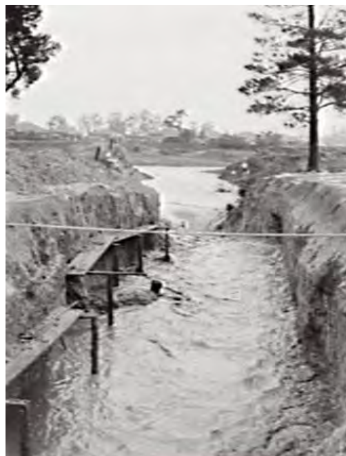
Stormwater Canal Construction 1932
