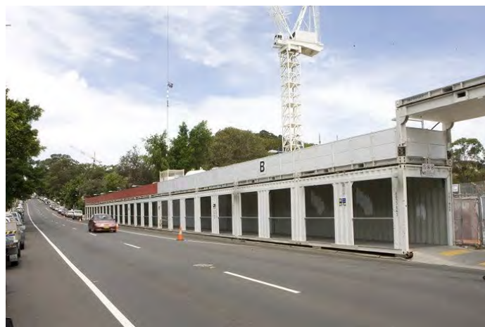
Image – Typical Type B Hoarding
