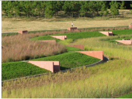
Figure 24: North Carolina Museum of Art detention basin converted to wetland (Source: surface678.com/north-carolina-museumof-art-pond-4 )
