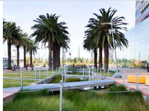
Figure 22: Melbourne Docklands - Overland flow path as a passive recreational space. (Source: www.aecom.com.au)
