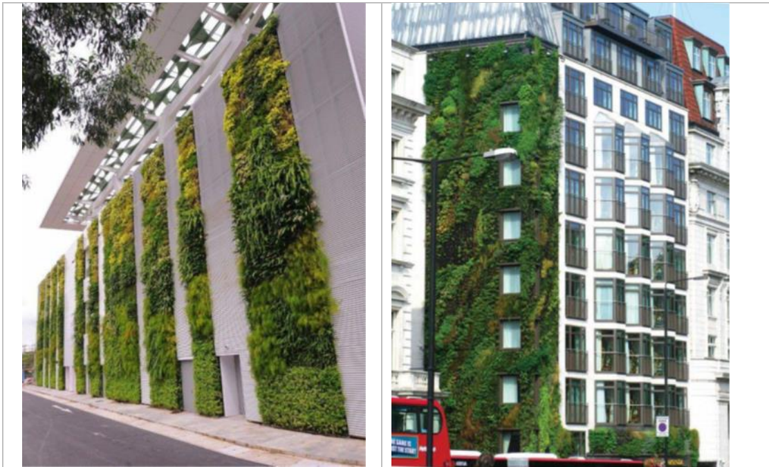
Figure 15: Biowall (green wall) (source: www.pinterest.com )
