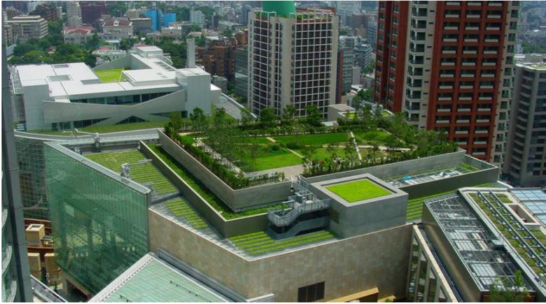
Figure 14: Roof garden (source: www.pinterest.com )
