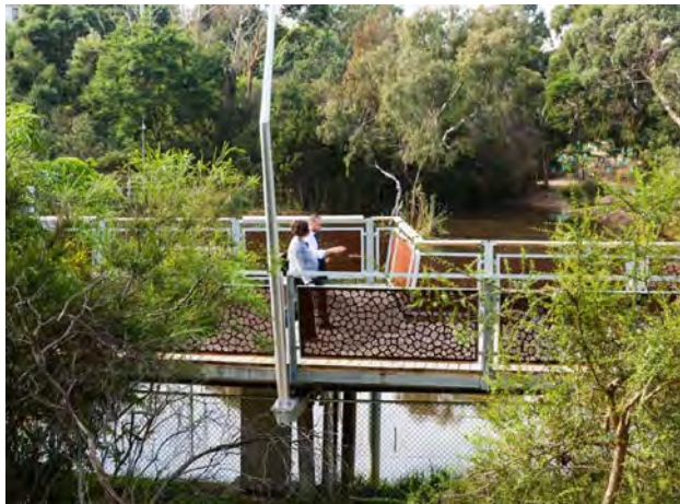
Figure 97: Elevated walkway at Jock Marshall Reserve and Nature Walk, Clayton, Victoria
