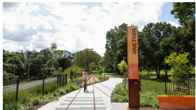
Figure 52: Informative maps and signage - Caboolture Wamuran Rail Trail
