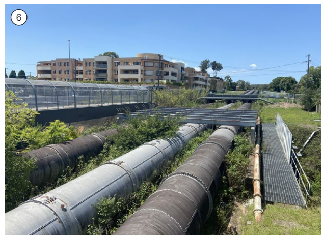
Figure 23: Supply pipes and road crossings at Regents Park
