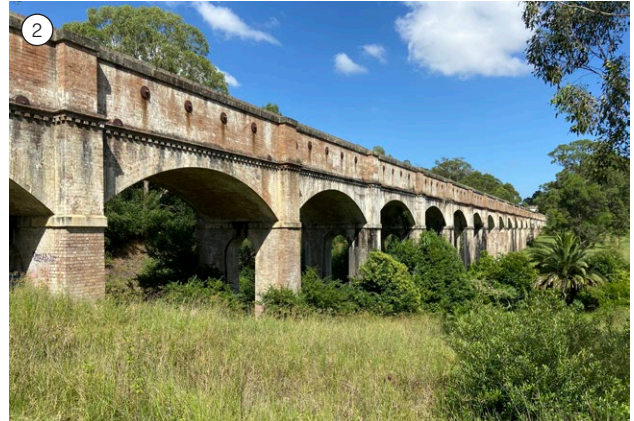
Figure 21: Corridor West - Boothtown Aqueduct, Greystanes
