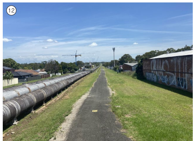
Figure 29: Land is cleared around the corridor where there is only private access
