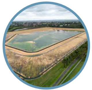
View south over Potts Hill Reservoir
