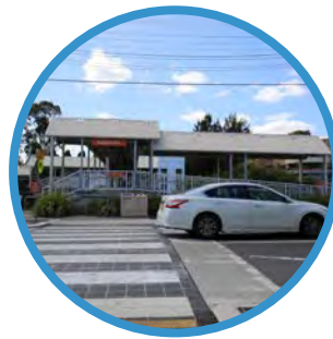
Park Road entry (west) to Regents Park Train Station
