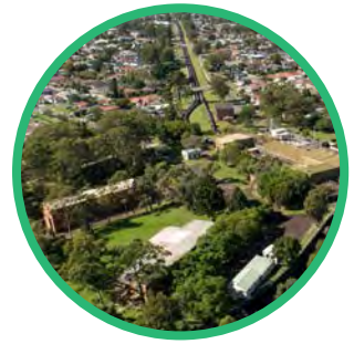
View south east over Guildford Pipehead Complex
