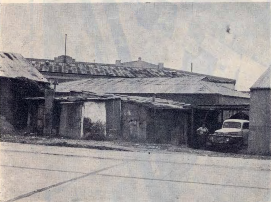
Some of the buildings demolished to make way for the new Civic Road and shops.
